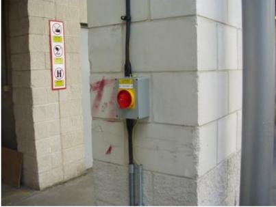
Barrel type switch – when the switch is turned to off two holes line-up and a padlock can be inserted to lock-off and prevent the switch being rotated and turned back on
