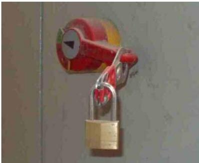
Main switch on a control panel at a recycling plant – padlock placed through switch preventing it being turned back on (note – a lock-off plate has been used here which allows more than one padlock to be used – see below)
